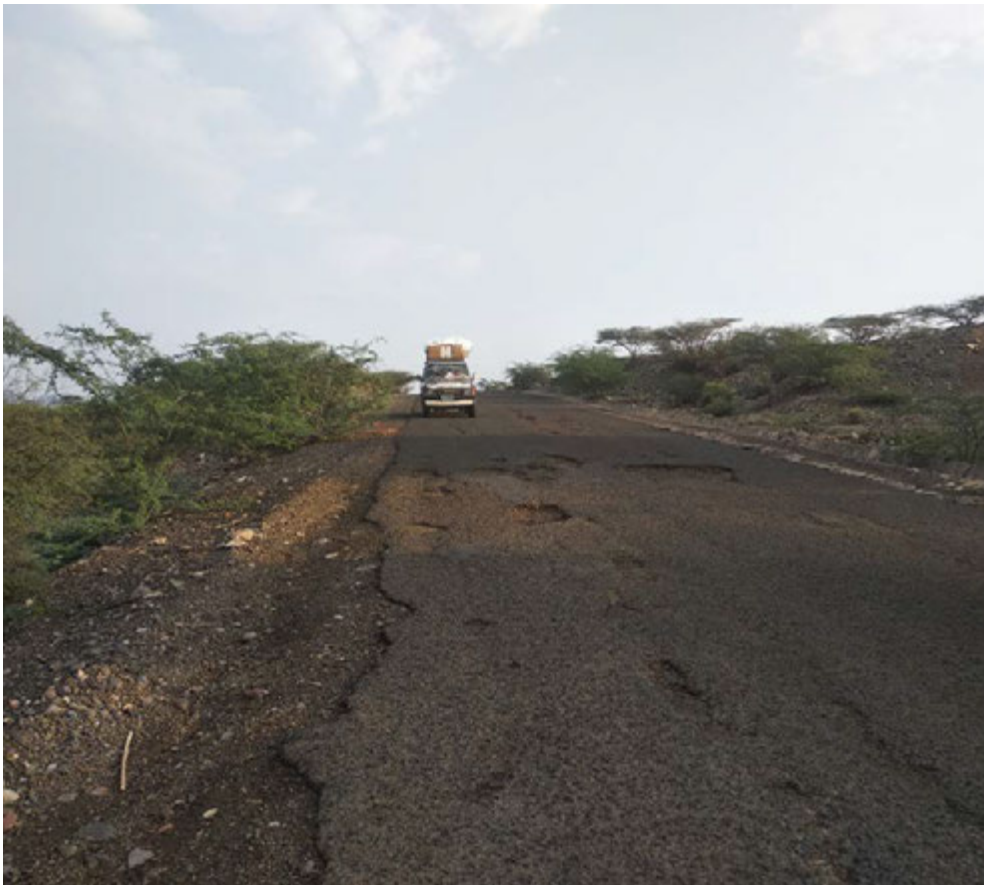
The asphalt part of Mokha Road to Taiz, full of potholes that cause traffic accidents for travelers. Al-Wazzaia - The road from Al-Khaleh to Taiz
