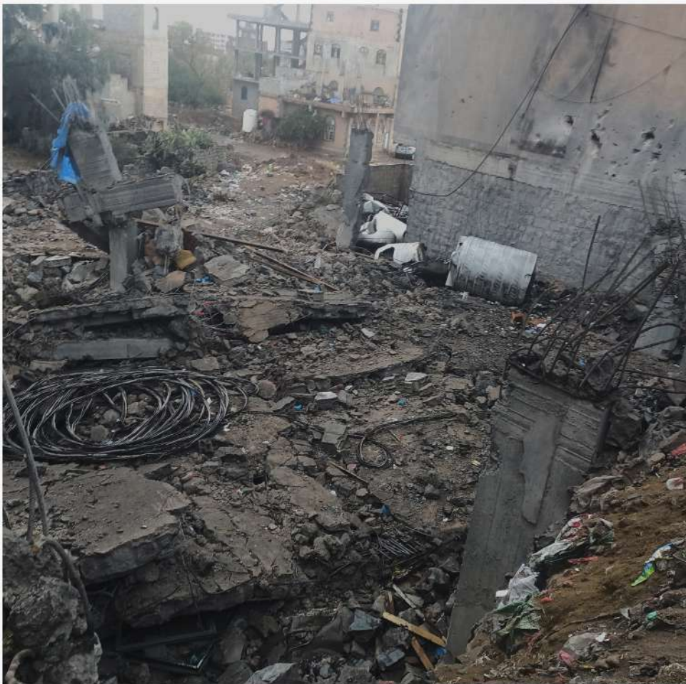
A second image of the incident site (a basement) in Sana'a City following US airstrikes under "Operation Rough Rider" on March 23, 2025.
