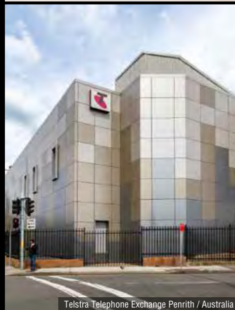
Telstra Telephone Exchange Penrith / Australia
