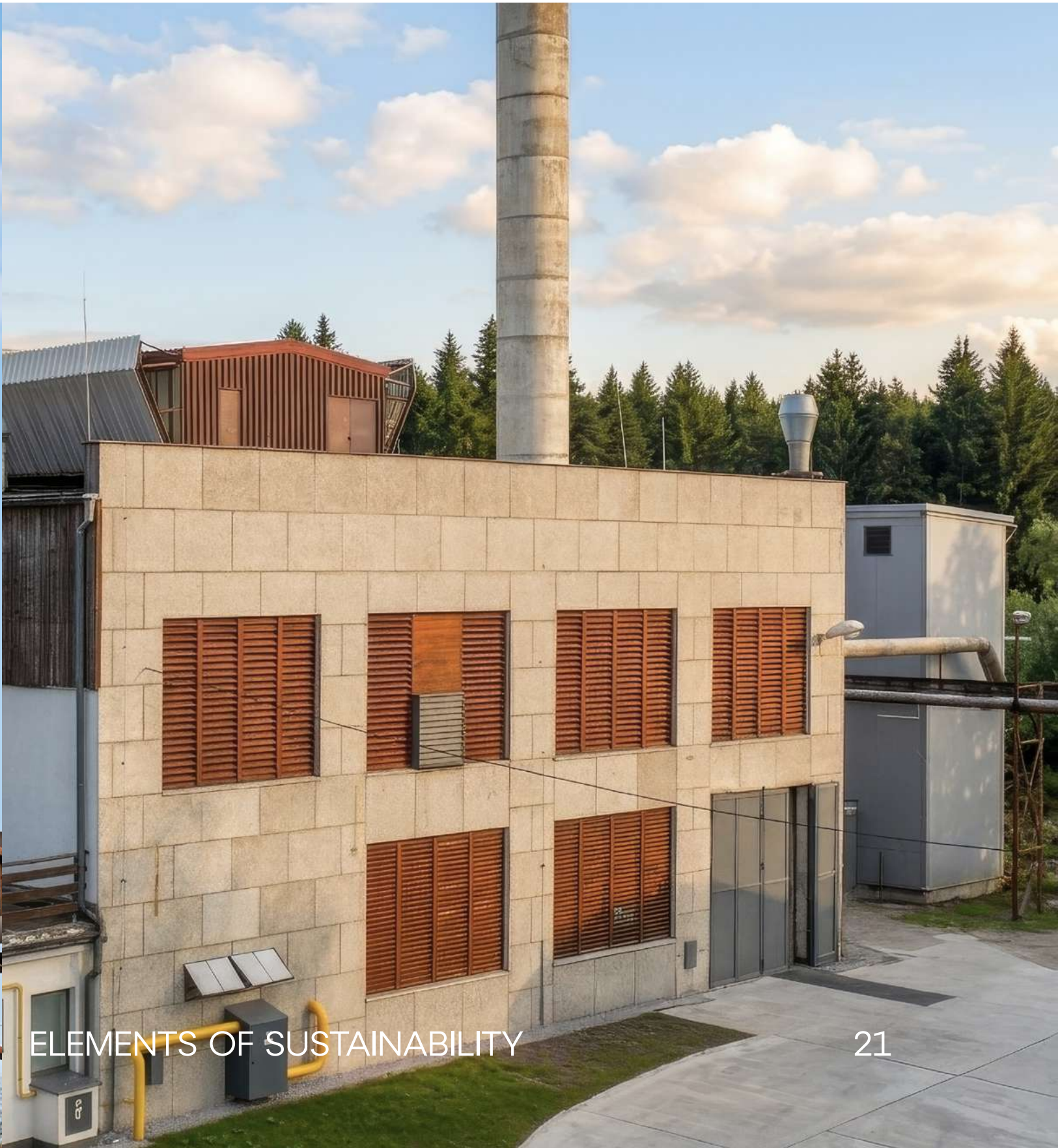
2024 INSULATION OF THE GLASSWORKS AND WINDOW REPLACEMENT
