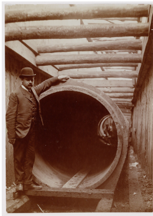
Sewer construction, Amsterdam, 1910–12. Copyright: Stadsarchief Amsterdam, CCo.
