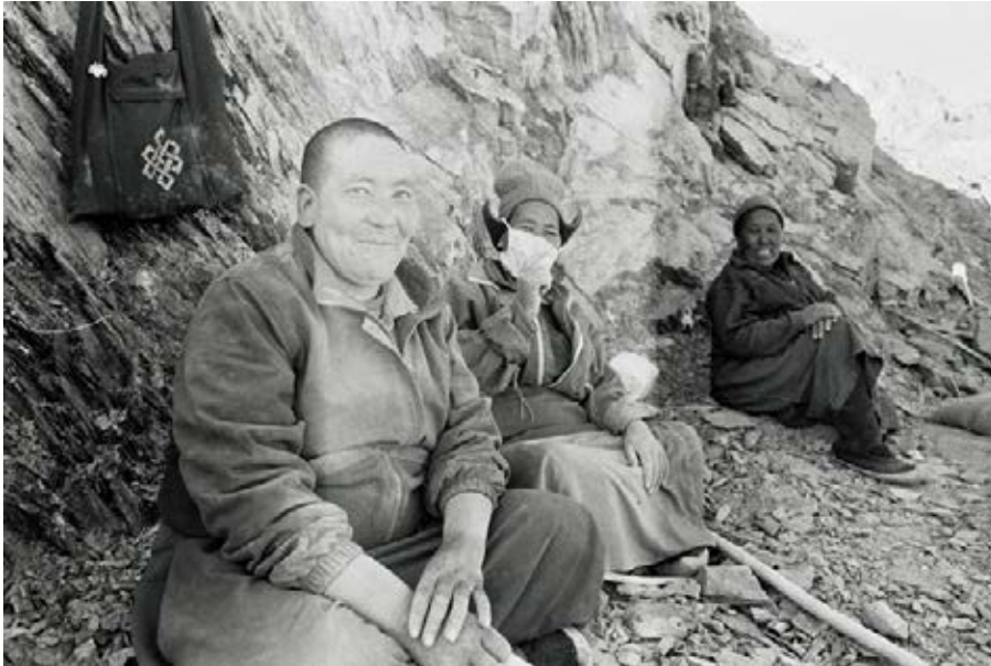
Ani Lobzang, Ani Angmo and Ani Kundzes take a break to sit down and rest on the road building site. Photo: Marta Normington
