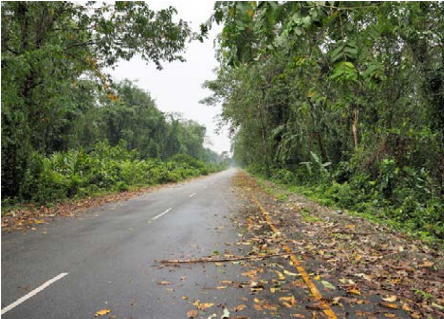
A pickled road, preserved for future connectivity. Photo: Edward Boyle.
