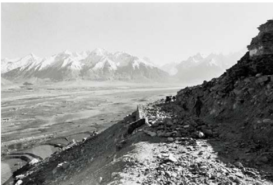
In the evening, after another day of work: the road in the process of being built.
