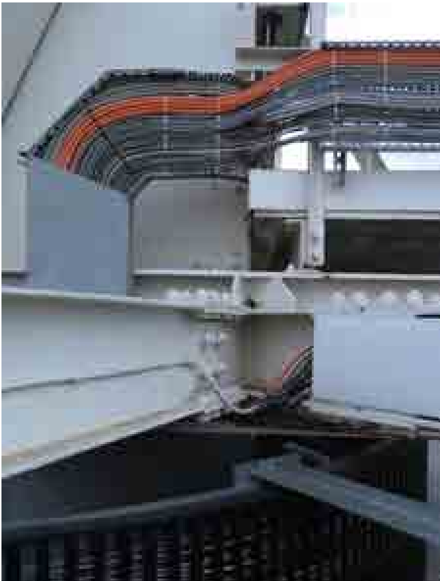
Cable wraps that transport data and power from the receiver to high-performance computers in the laboratory below.
