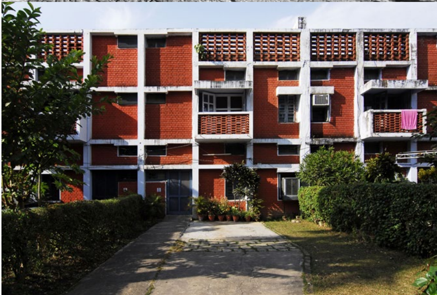
Maintenance of the Chandigarh-Style, referred to as "straight line" by residents. The availability of hand-made bricks and the climatic conditions (temperatures, wind and monsoon) led to purist design principles.
