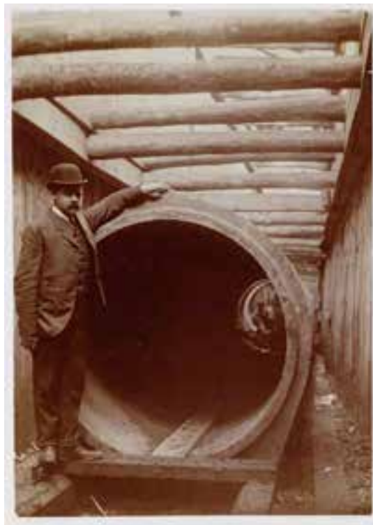
Sewer construction, Amsterdam, 1910–12. Copyright: Stadsarchief Amsterdam, CCo.
