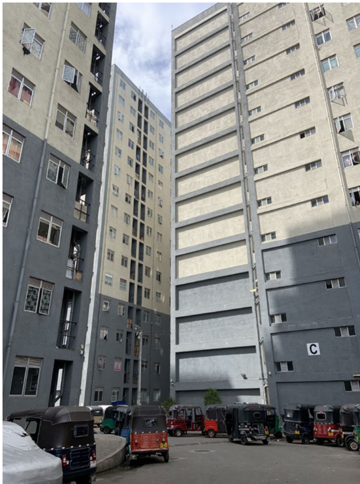
Car parks and balconyless concrete buildings.
