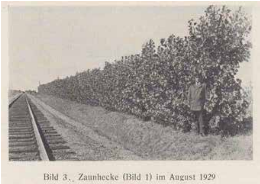
Test strip of Wiechula's snow fence along the railway line in Barleben near Magdeburg, 1929. Renz 1930: 86.
