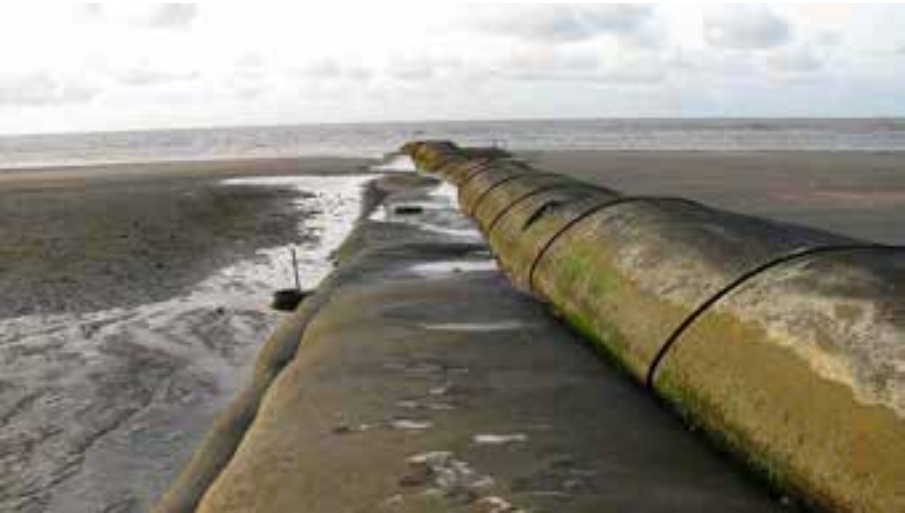
← Typical soft groyne in Guyana.
