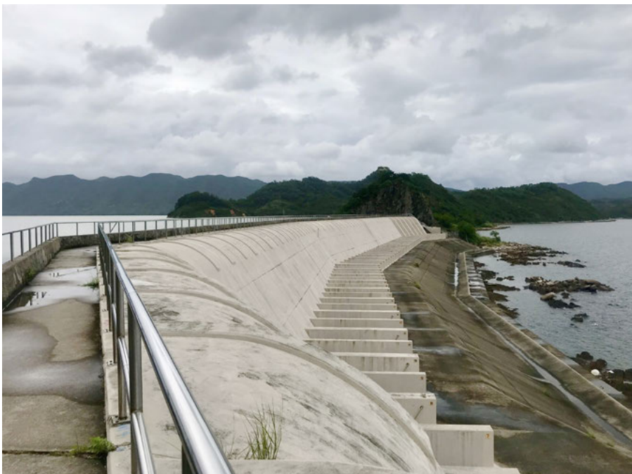
Concrete sub-dam, Plover Cove Reservoir, Hong Kong. Photo: Natalia Echeverri, 2020.
