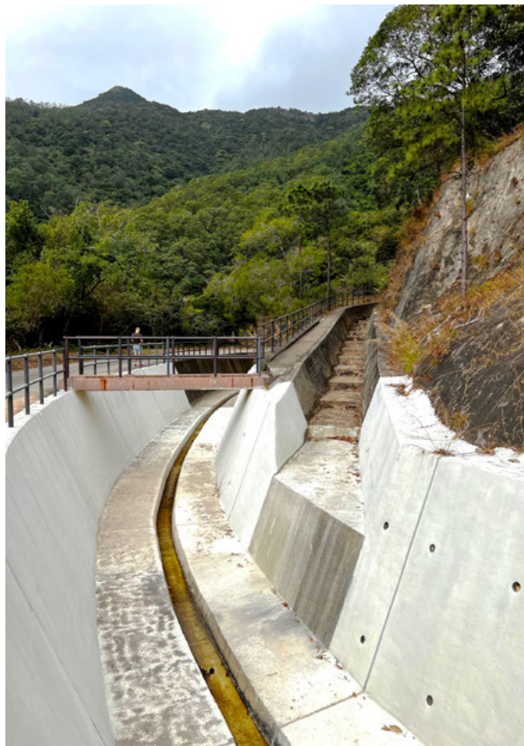
Catchwater with secondary stepped channel next to the Southern Lantau trail during the dry season. Photo: Natalia Echeverri, 2024.
