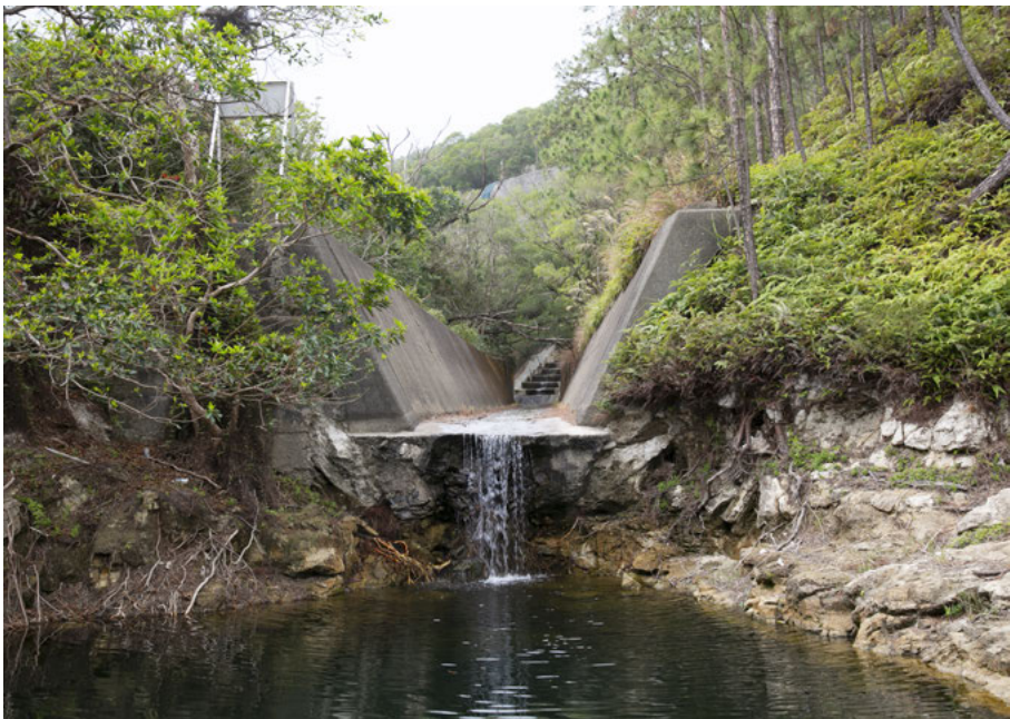
Shek Pik catchwater discharge into the reservoir during the dry season.
