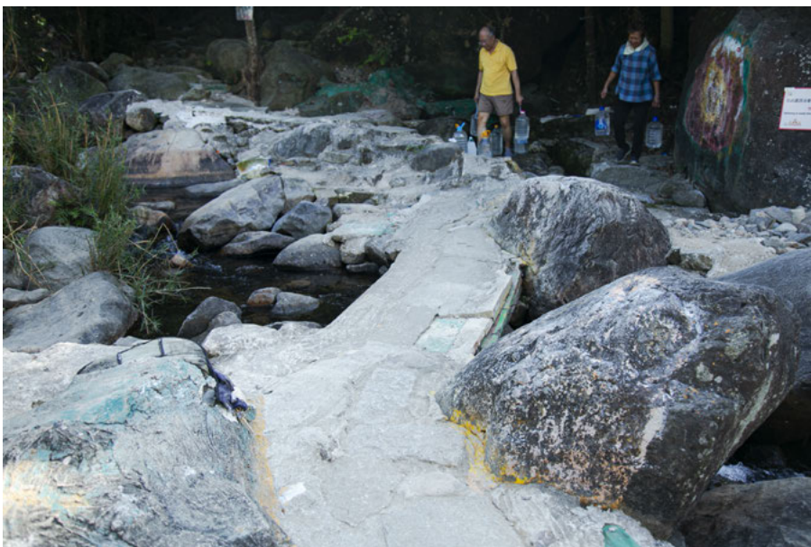
Bridge made from a wood span and layers of topping cement supports a steady traffic of local residents carrying bottles filled with fresh water.
