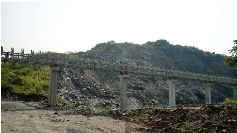
A conveyor belt moves stone from a quarry to a cement factory below, Kaeng Khoi, Saraburi. Photo: Eli Elinoff, 2019.
