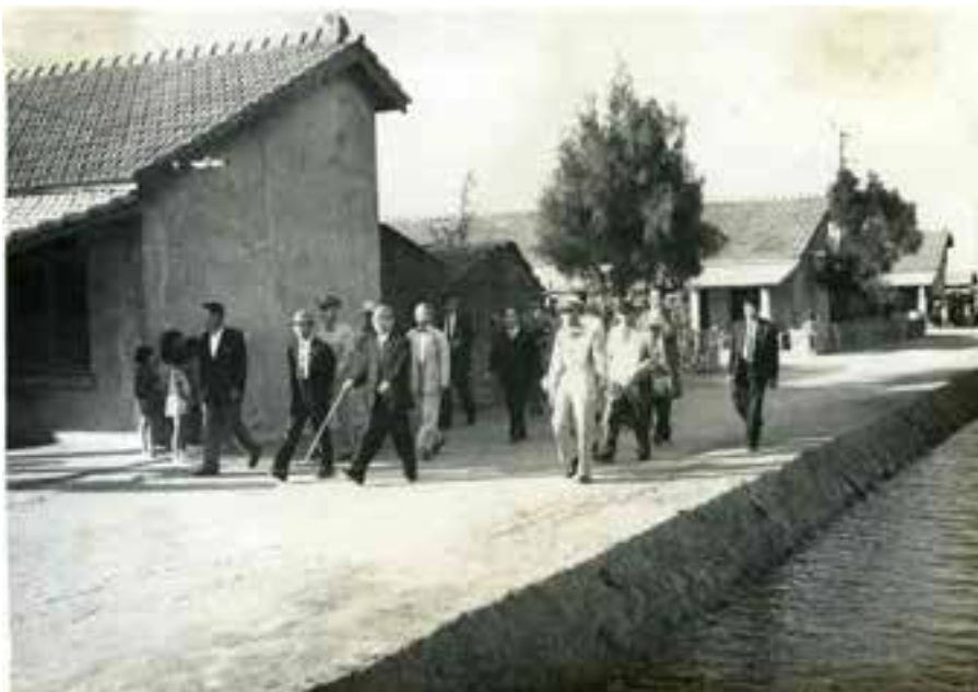
SWH housing at Budai Saltworks.
