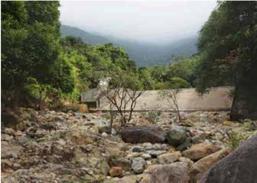
22-meter-wide dam with a linear intake intercepts the Wong Lung Hang Stream, leaving a rocky streambed exposed.
