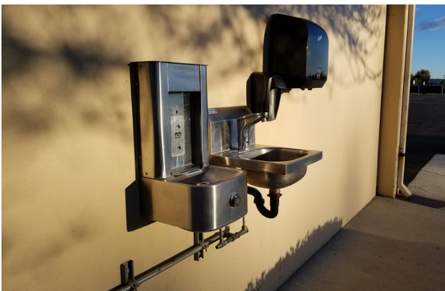
A newly installed filtered water bottle-filling and handwashing station at Azusa High School. Photo: Fred Ariel Hernandez, 2023.
