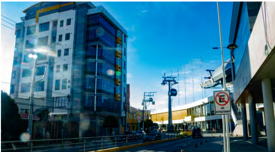
Station building of the Yellow Line of Mi Teleférico. Photo: Herland Jarro Arteaga, El Alto, August 2020.
