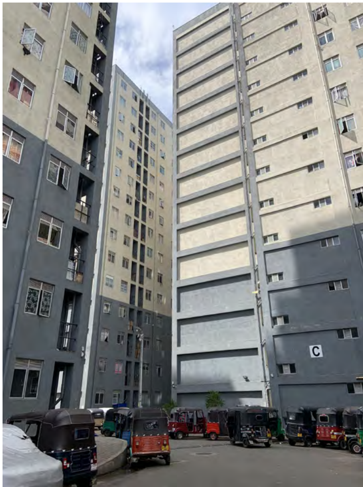
Car parks and balconyless concrete buildings.
