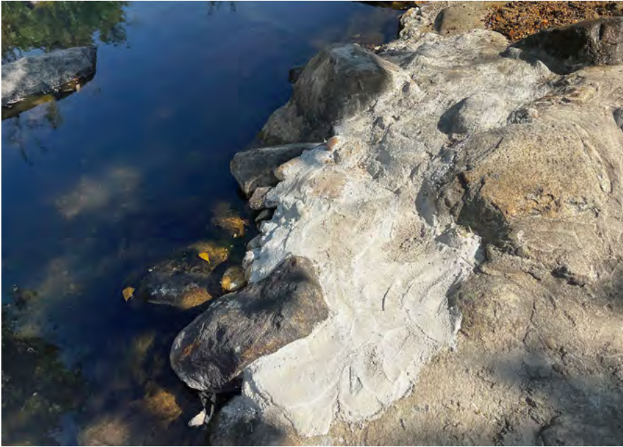
Recently cast concrete texture constructed by Filipina domestic worker who uses concrete to flatten and prevent erosion of a gathering area.
