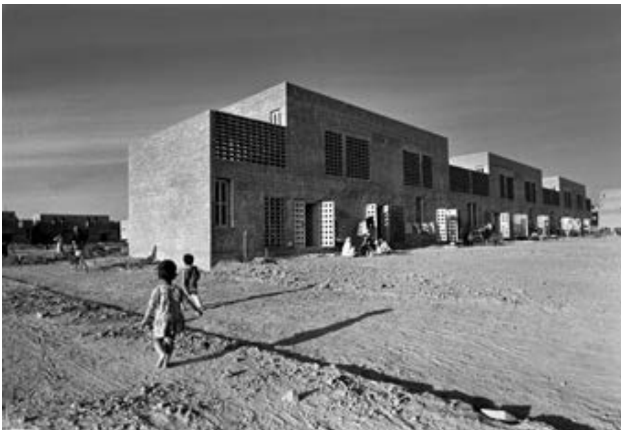
Early government housing in 1968, designed by Jeanneret, who lived as first chief architect in Chandigarh for fifteen years, and the British architect couple Fry and Drew who stayed from 1951 to 1954.
