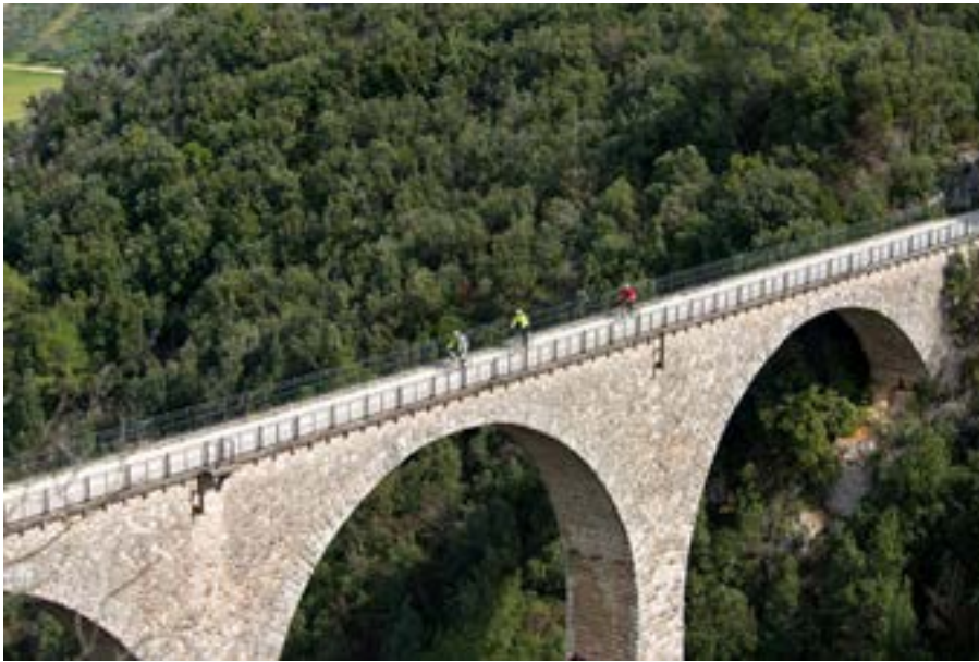
Cycling on the Caprareccia viaduct along the decommissioned Spoleto–Norcia railroad line.
