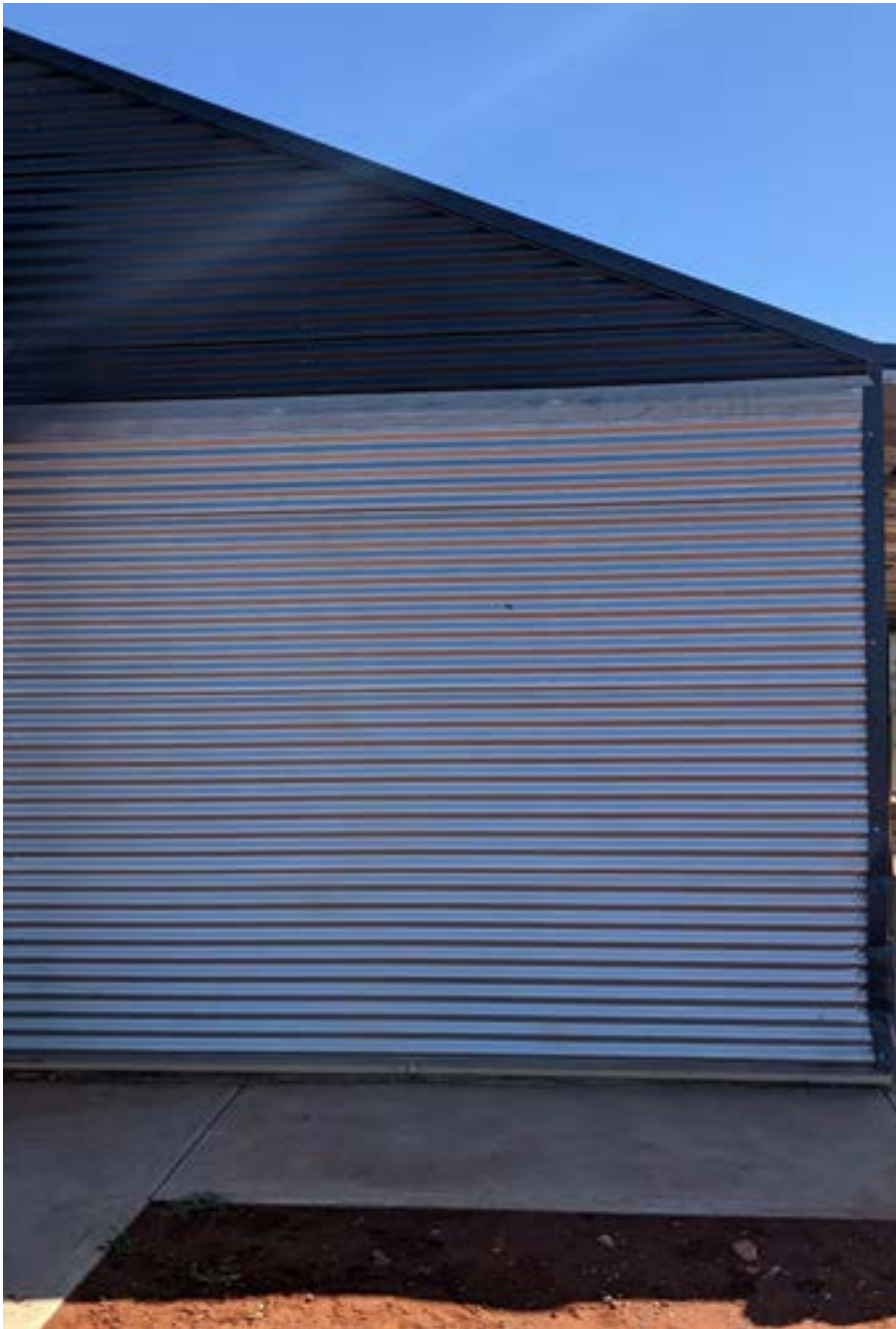
A perforated Zincalume custom orb skin is attached to the external wall of this new house on the APY Lands in order to reduce internal temperatures.
