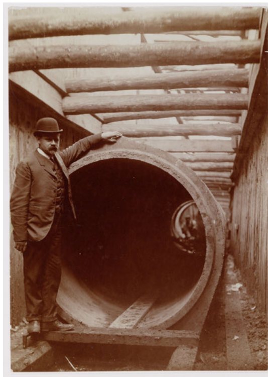
Sewer construction, Amsterdam, 1910–12. Copyright: Stadsarchief Amsterdam, CCo.
