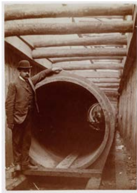
Sewer construction, Amsterdam, 1910–12. Copyright: Stadsarchief Amsterdam, CCo.
