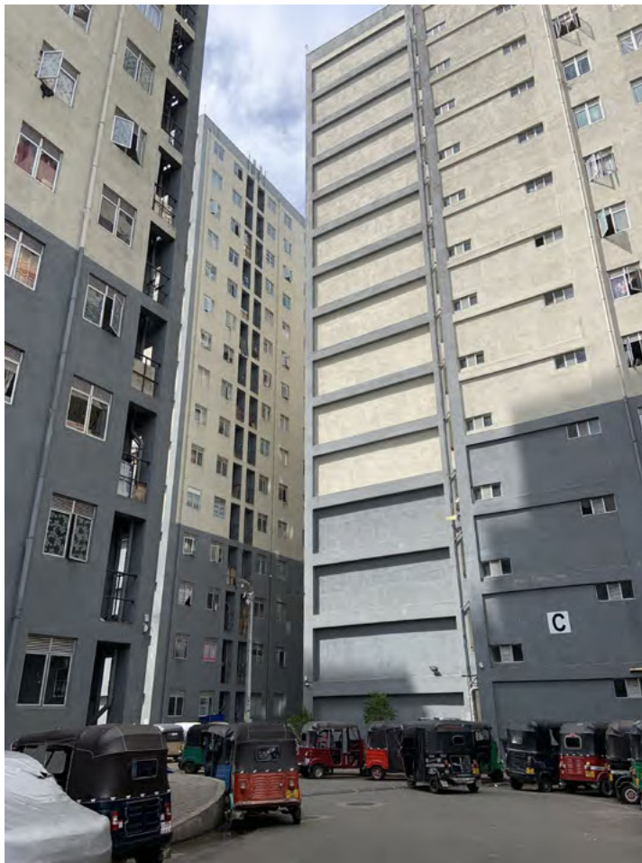
Car parks and balconyless concrete buildings.
