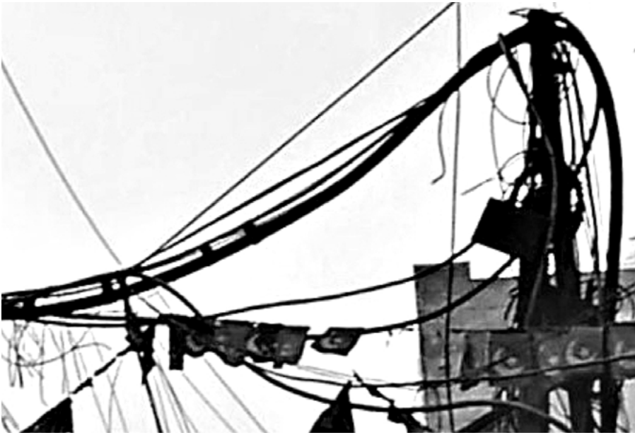
A Meshwork of Wires. Hooking onto the grid via improvised connections. Photo: Maan Barua, 2020.
