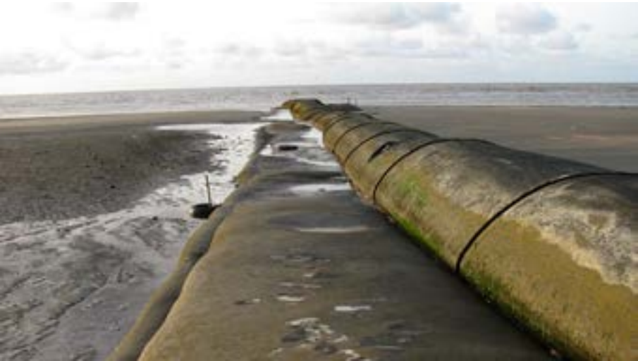
← Typical soft groyne in Guyana.
