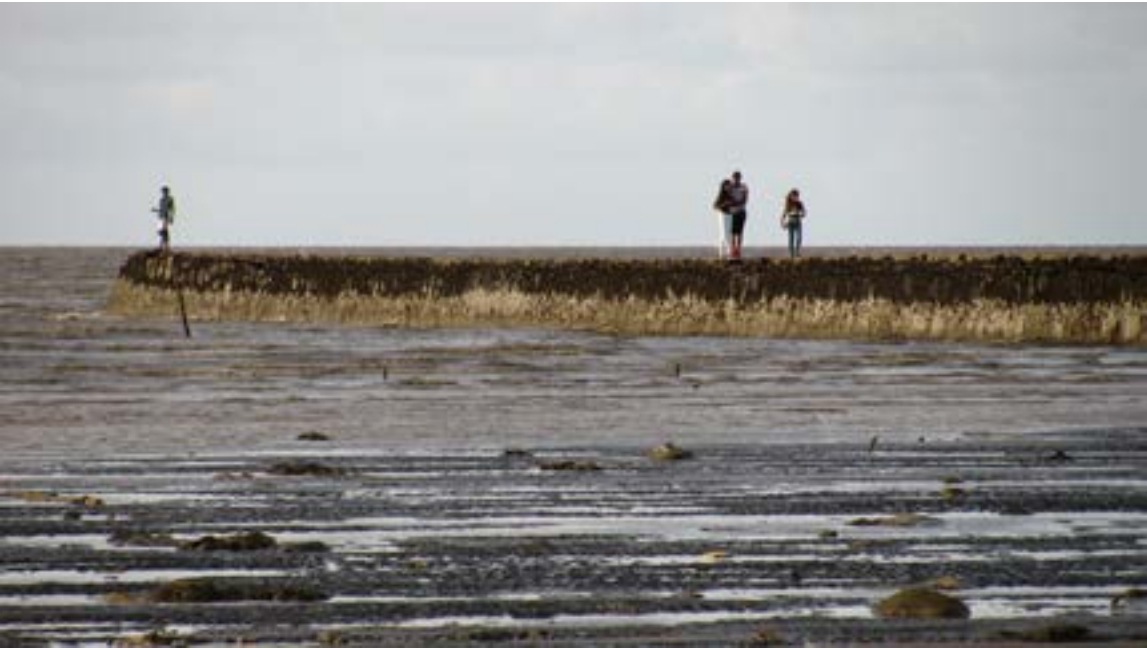
↓ A typical concrete groyne in Guyana. Photo: Sarah E. Vaughn, 2014. ↓↓ Fisherman mending a net. Photo: Sarah E. Vaughn, 2014.
