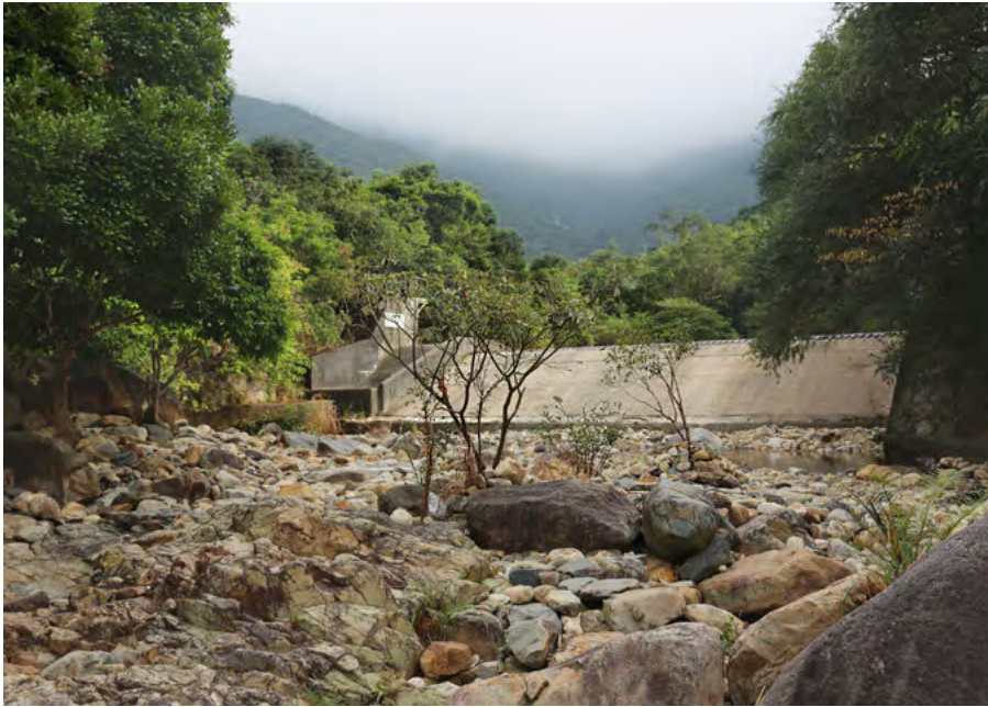
22-meter-wide dam with a linear intake intercepts the Wong Lung Hang Stream, leaving a rocky streambed exposed. Photo: Natalia Echeverri, 2023.
