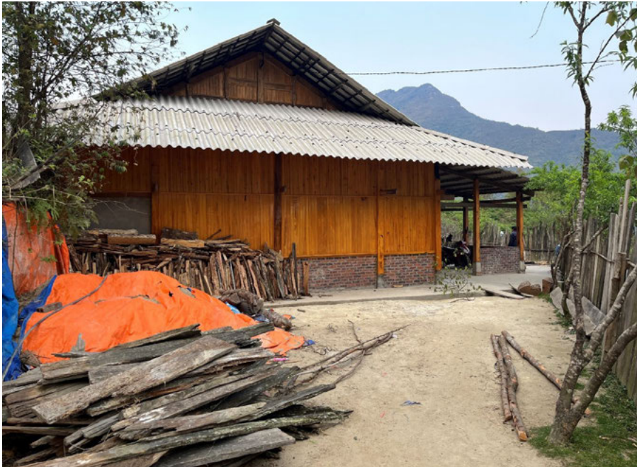
New Hmong house on a concrete slab with low brick walls, Seo Mi Ty Commune, Sa Pa District, Lào Cai Province. Photo: Authors, 2023.
