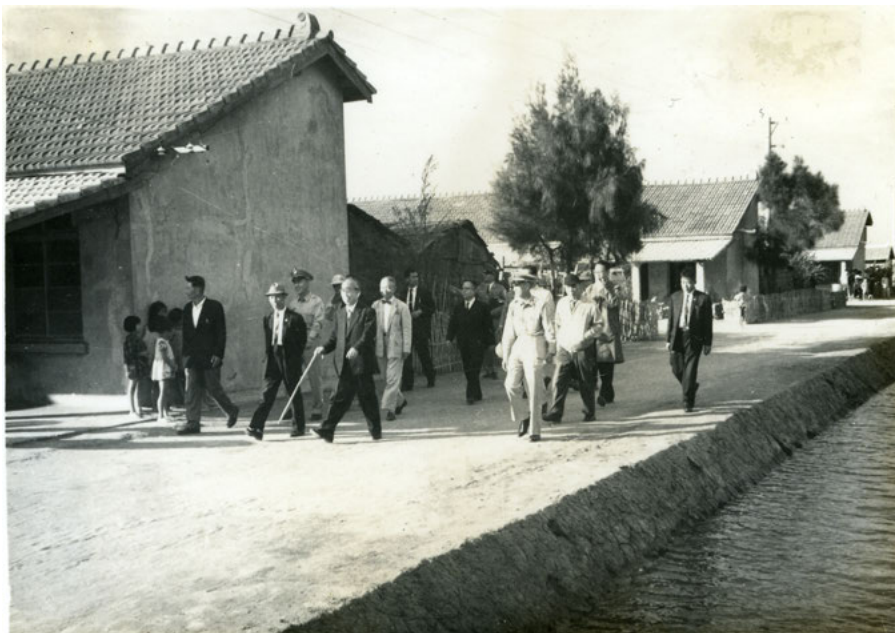
SWH housing at Budai Saltworks.
