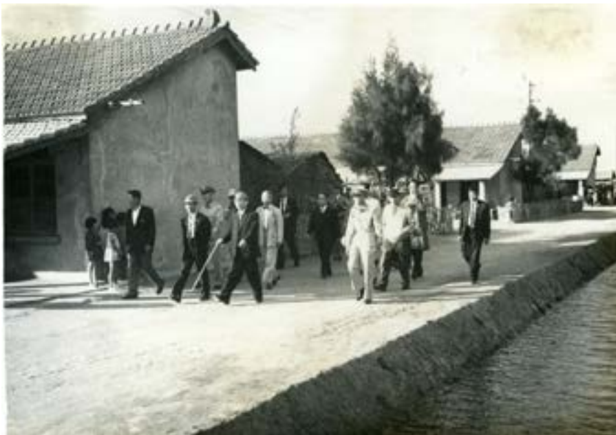
SWH housing at Budai Saltworks.
