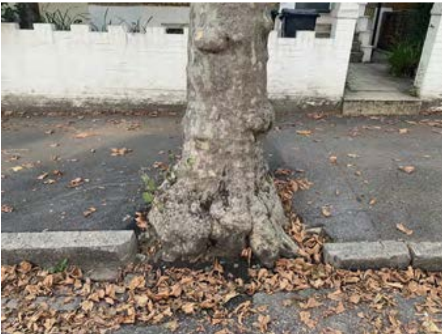
A curb is removed to make space for an expanding tree, London.
