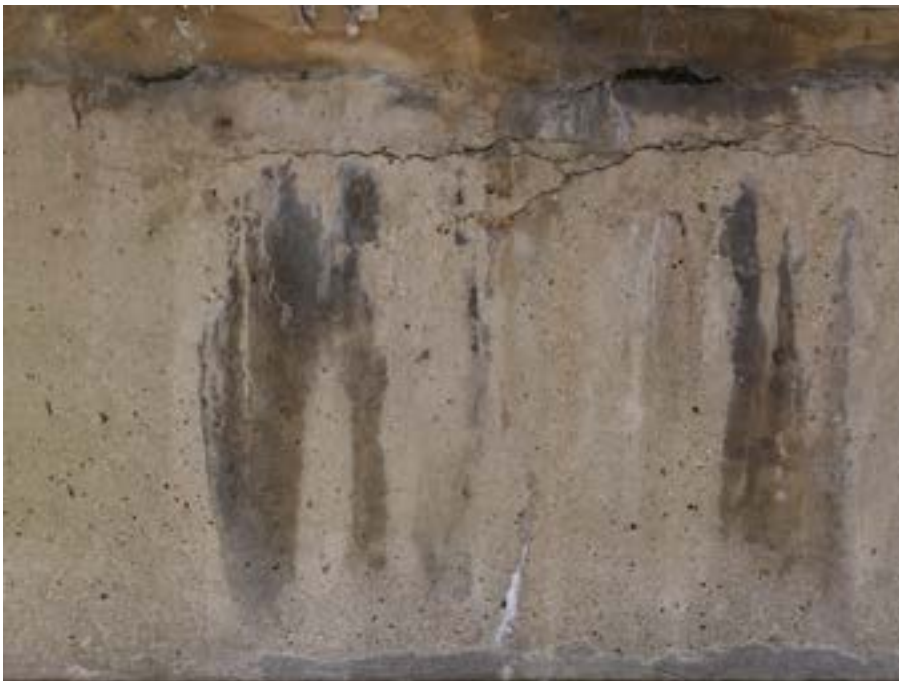
Concrete as microbiome. The darker patches contain cyanobacteria. Bedford Way, London. Photo: Matthew Gandy, 2021.
