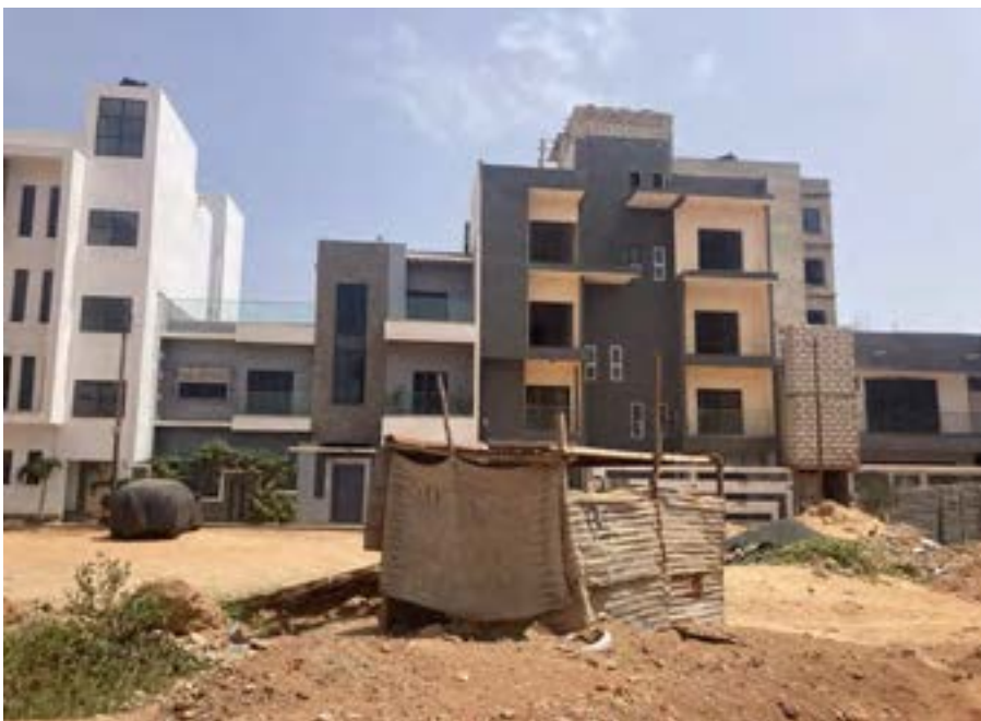
Global aesthetic of concrete in Dakar, Senegal. Photo: Pierre Wenzel, 2023.
