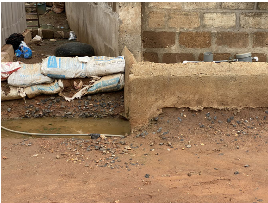
Sand and nylon bags used to construct flood barriers in the upmarket and upstream neighbourhood of East Legon, Accra. Photo: Afra Folli, 2020.
