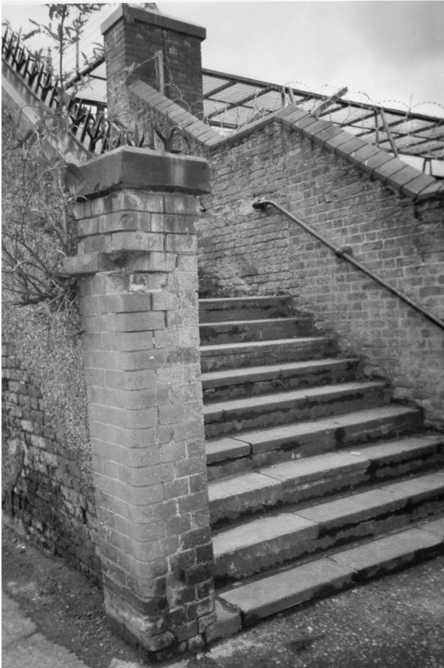
Stairs to railway bridge linking Lansbury Estate and Teviot Estate. Photo: Jimmy Watters, mid-1990s.
