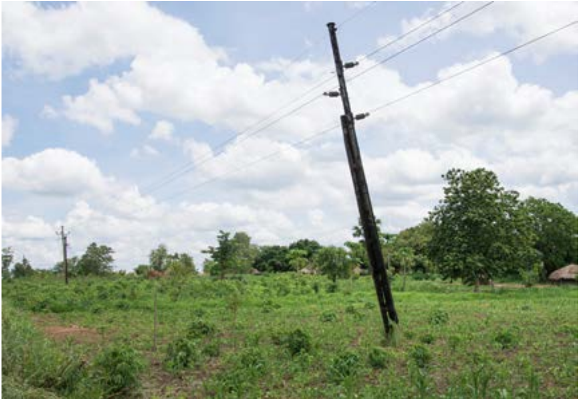
↑ A broken electricity pole that has been provisionally repaired leans dangerously over a field.
