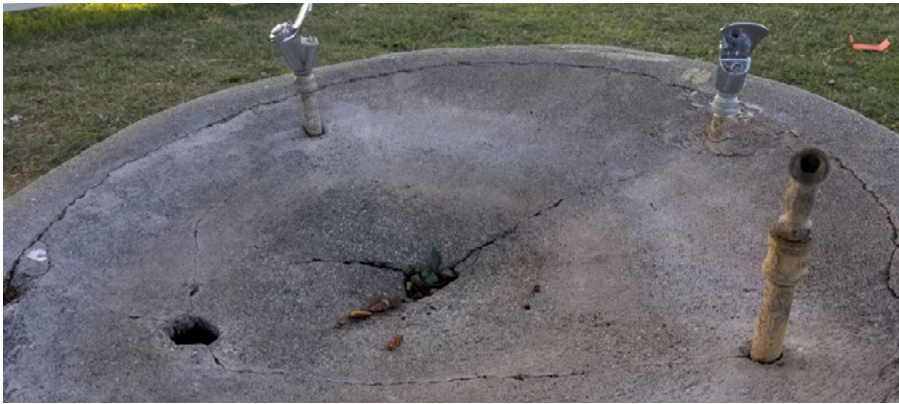
Aging concrete water fountain near the sports fields at AHS. Plant matter collects in the center. Two spigots function, one is missing, another rusted. Photo: Fred Ariel Hernandez, 2022.
