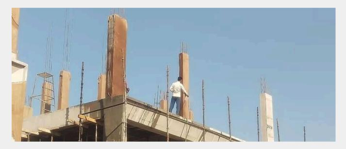
18 villas have completed all slab work, with brickwork and internal plastering in progress.
