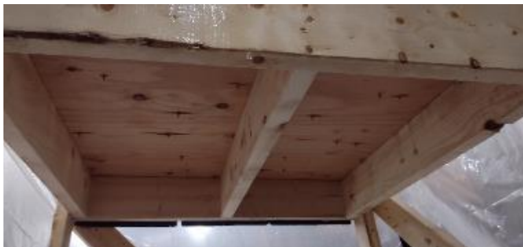
Photo No. 2 SunStack (SSB1) Solar Mount, Bottom View
