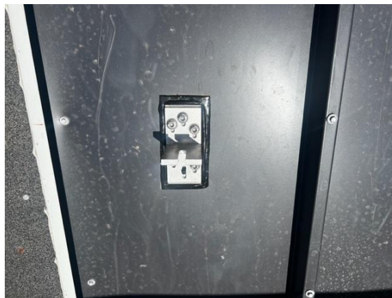
Photo No. 6 Typical SSM Metal Roof Installation
