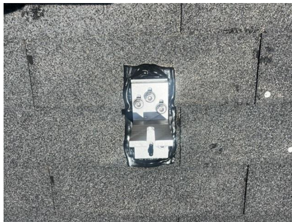
Photo No. 4 Typical SSM Asphalt Shingle Installation
