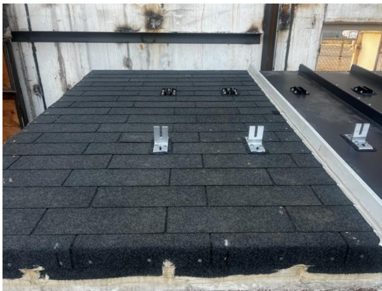
Photo No. 1 Asphalt Roof Shingle Install
