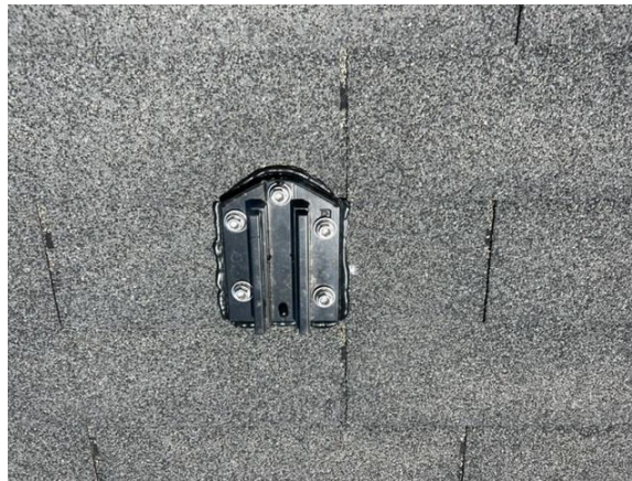
Photo No. 3 Typical SSB1 Asphalt Shingle Installation
