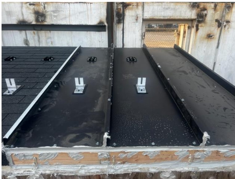
Photo No. 2 Metal Roof Install
