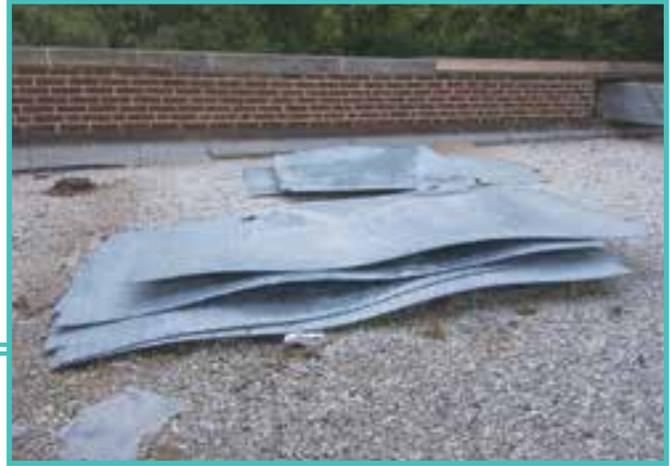
FIGURE 17: DISTORTION (ACCEPTABLE)
