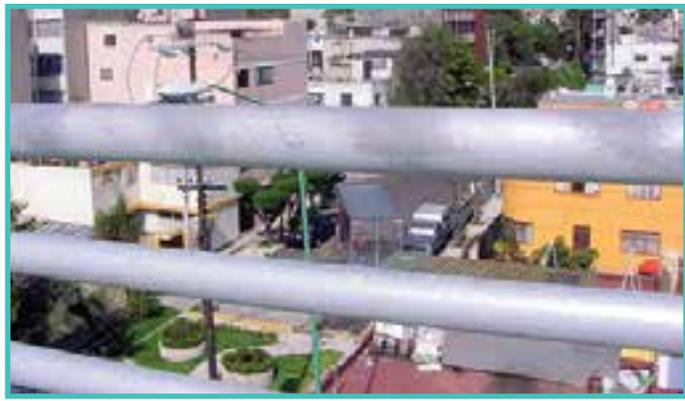
FIGURE 11: GRAY COATING DUE TO PROCESSING (ACCEPTABLE)
