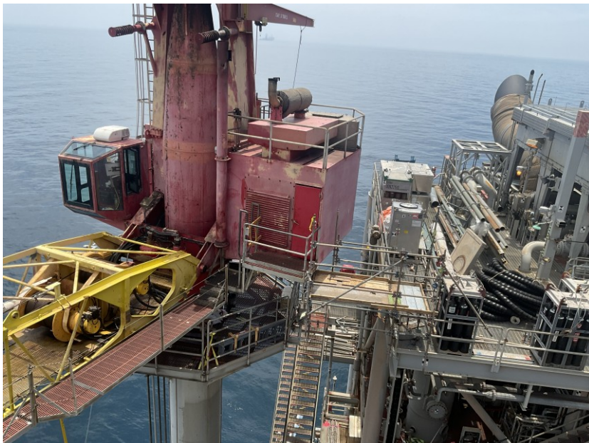
Bird's eye view of crane
