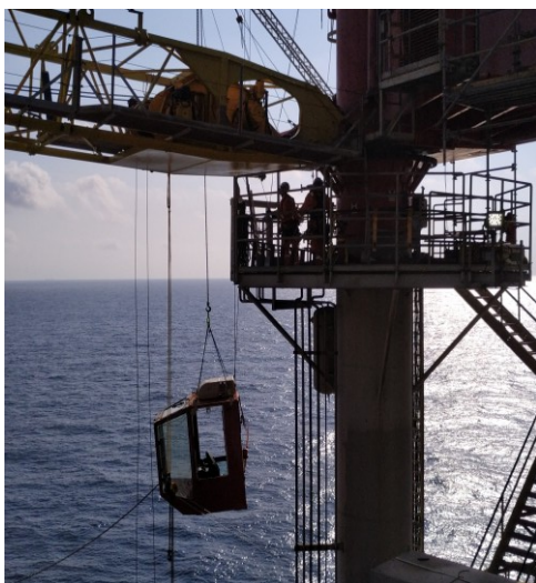
Lifting operation of crane cabin
