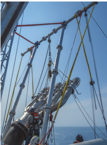
Installation of the new flare tip
