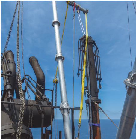
Removal of the old flare tip
