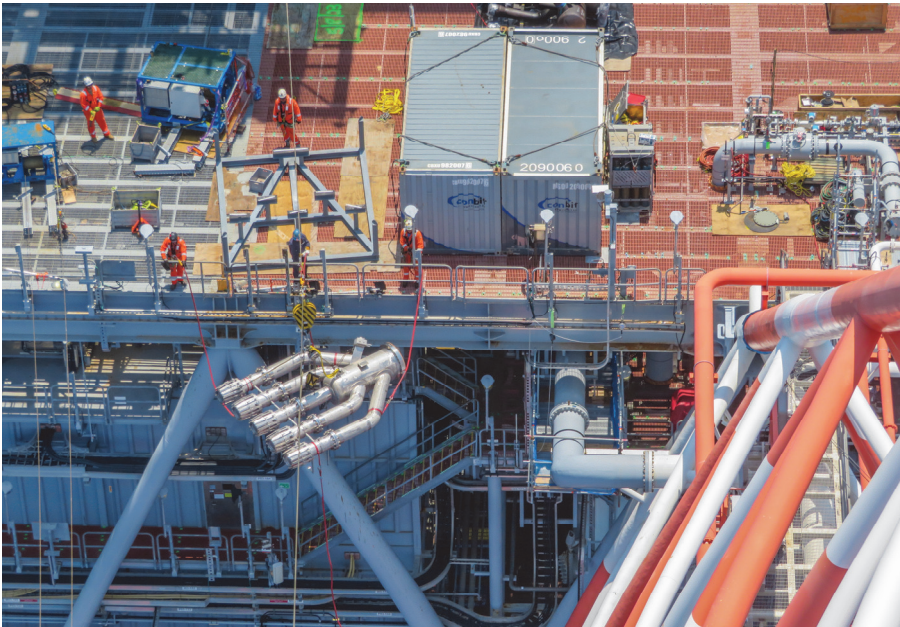
Lifting the new flare tip up to the flare tower
