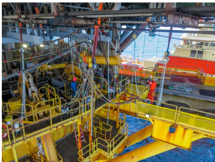
Rigging equipment lifting cylinder into position
