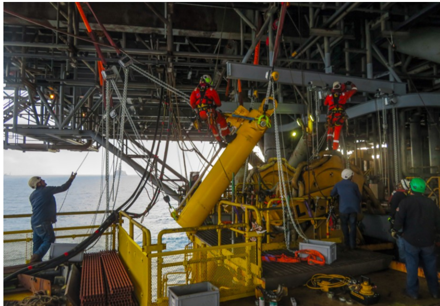
Rope access technicians installing cylinder into final position
