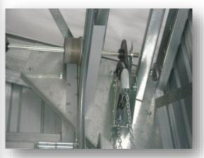
Widespan doors can be used in a wide range of applications including Aircraft/ Helicopter hangers, industrial and commercial structures. Each door is custom built to each individual door opening. Sectional doors are made up of individual sections with structural bracing, each section is guided by wheel inside a track section. Operation is either by manual hand chain or electric motor.
