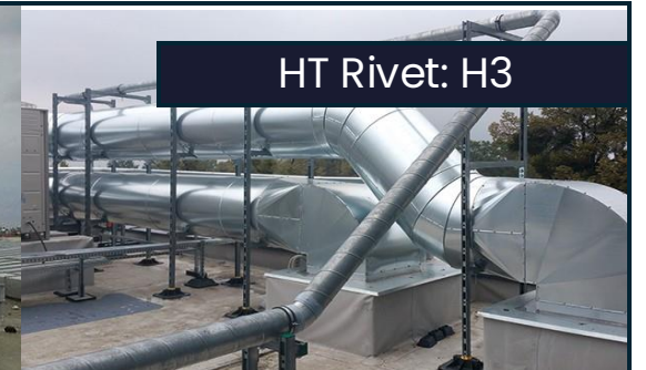
Ventilation Ducting & Support Frames
