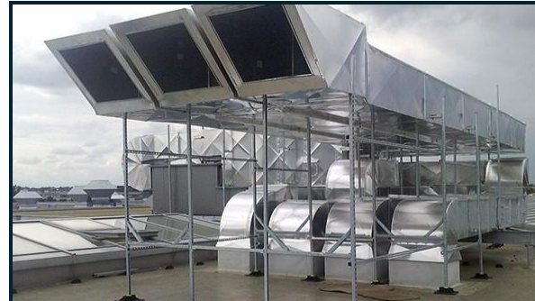
Ventilation Ducting & Support Frames
