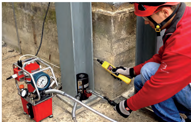
Foundation bolt connection.
