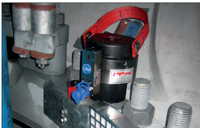
Tower bolt connection.
