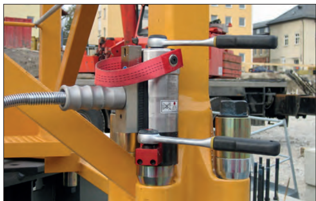
Tower segment bolt connection at tower crane.
