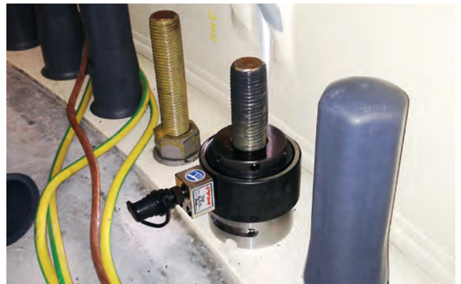
Foundation bolt tensioning.
