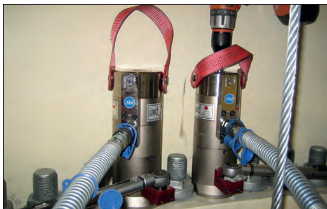
Tower segment bolt connection at wind turbine.
