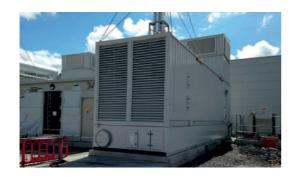
Our tanks are designed to accommodate up to 74 tonne acoustic housings on top of the tank and provide you with a 48HR cycle of product for generator run times. The design of this system is produced to reduce area needed on site and support the weight of the generator and all of its components.
