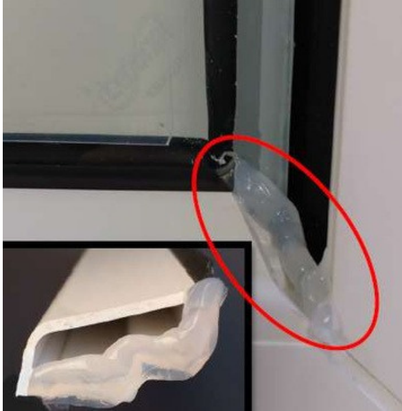
Fig. 3 Add neutral-cure silicone sealant
