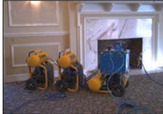
Figure 5. Dry fog system staged for treatment
