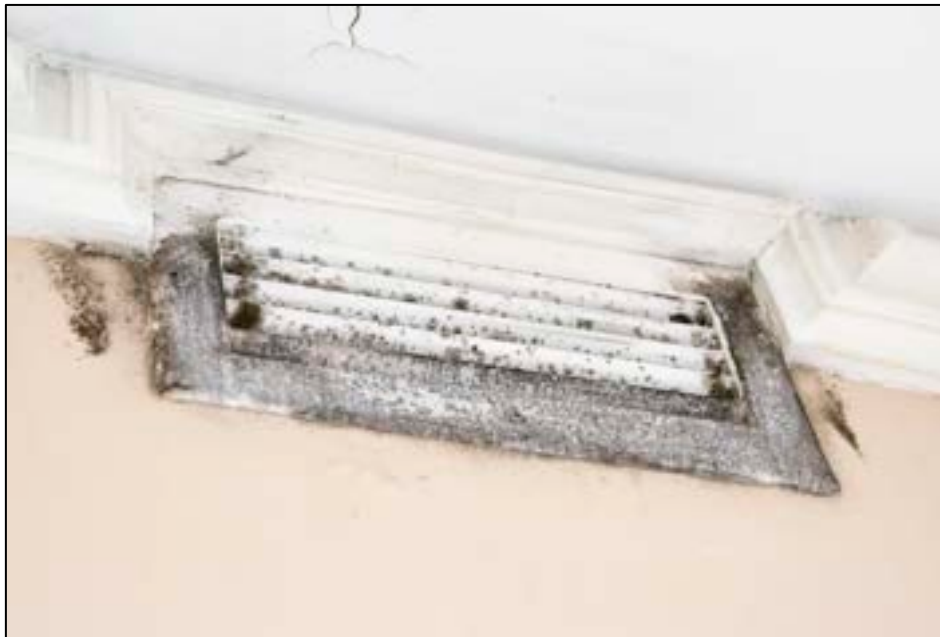
Figure 4. Mold/fungal growth at heat vent in Building 60
