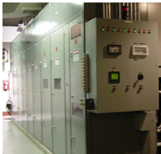
MV Equalizer system in a hospital, USA
