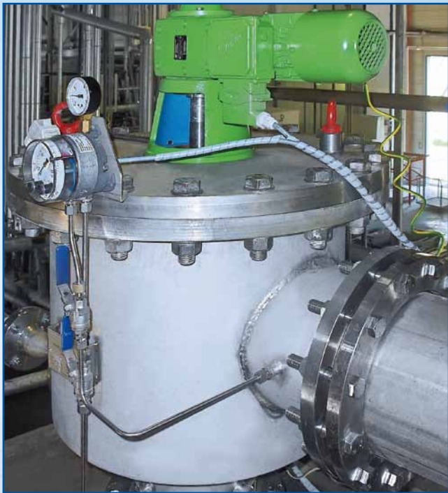
Fig. 8 cooling water filtration in plastics industry
