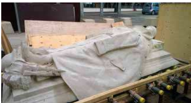
Fig 13 The catafalque cleaned and with initial nanolime treatment on its cradle ready for re-hoisting. Further treatment was carried out after it was lifted back into position.
