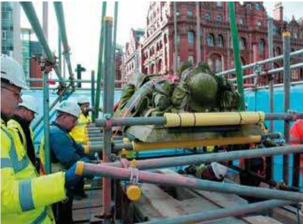
Fig 16 Lifting the catafalque from its bed on slings
