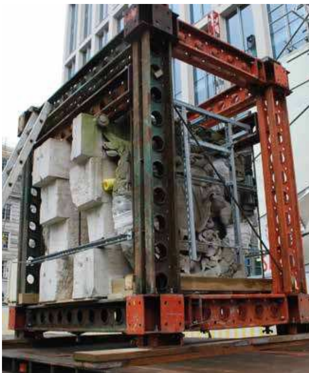
Fig 14 Removal of the fragile wreaths and coats of arms as a single assembly held together with clamps
