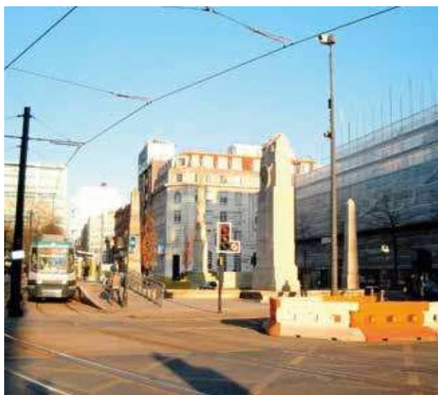
Fig 1 The tram stop in St Peter's Square, incorporating part of the cenotaph plinth, and general view of the setting
