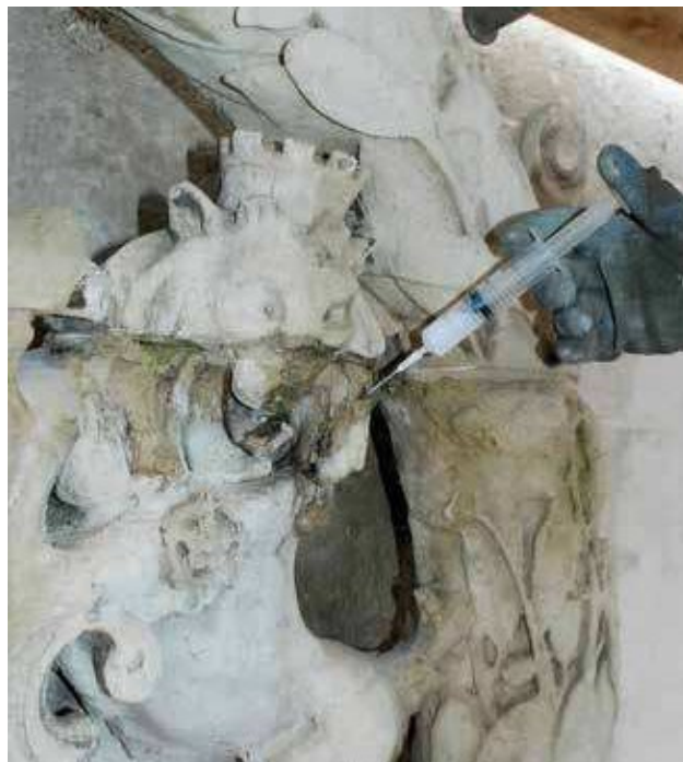
Fig 15 Nanolime and intricate repairs/stabilisation to the wreaths: replacement elements were carried out in lime/stone dust to maintain weather-proofing and aesthetic integrity with no re-carving or substantial piecing-in.
