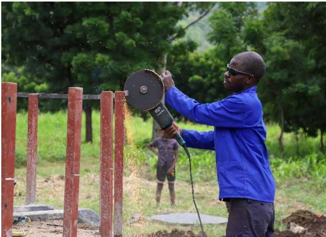
■ Figure 12: Installation of guard rails
