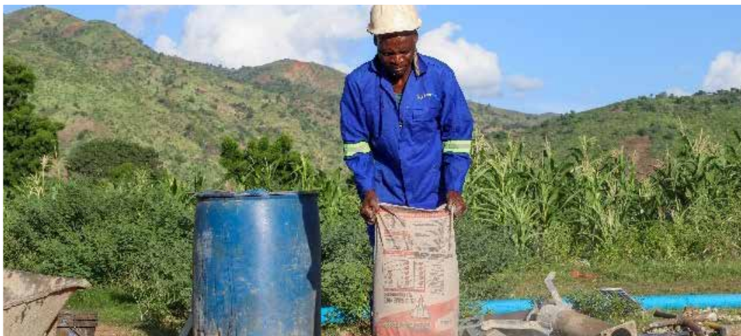
Figure 4: Site preparation works around the base of handpump - Excavation
