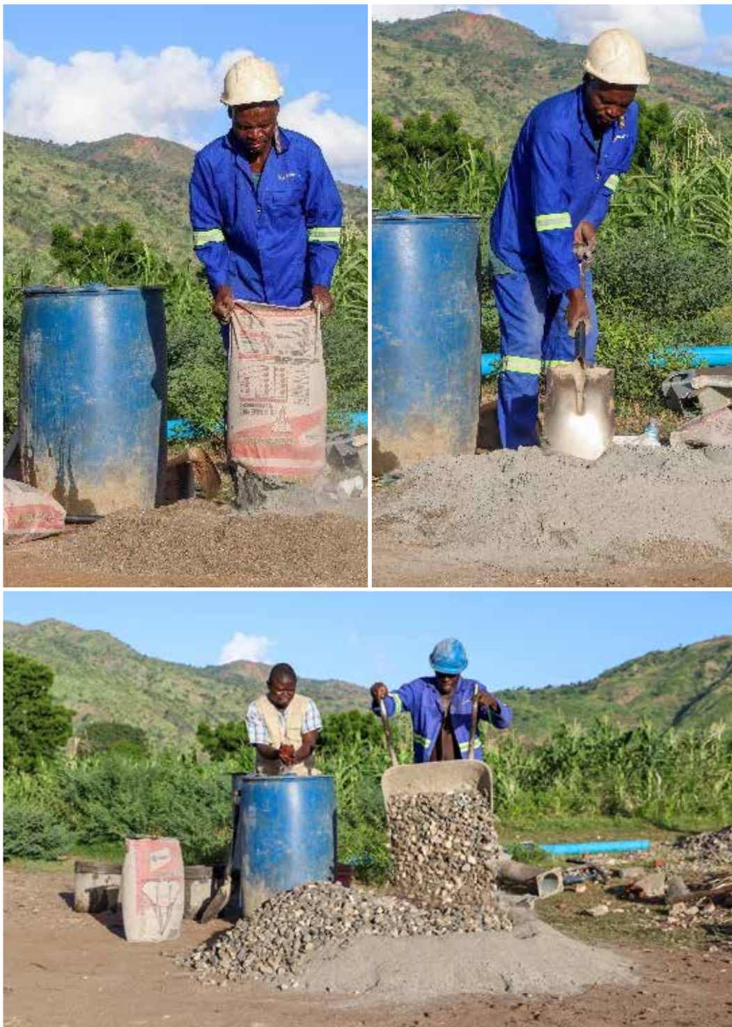
■ Figure 5: Mixing of concrete on site
