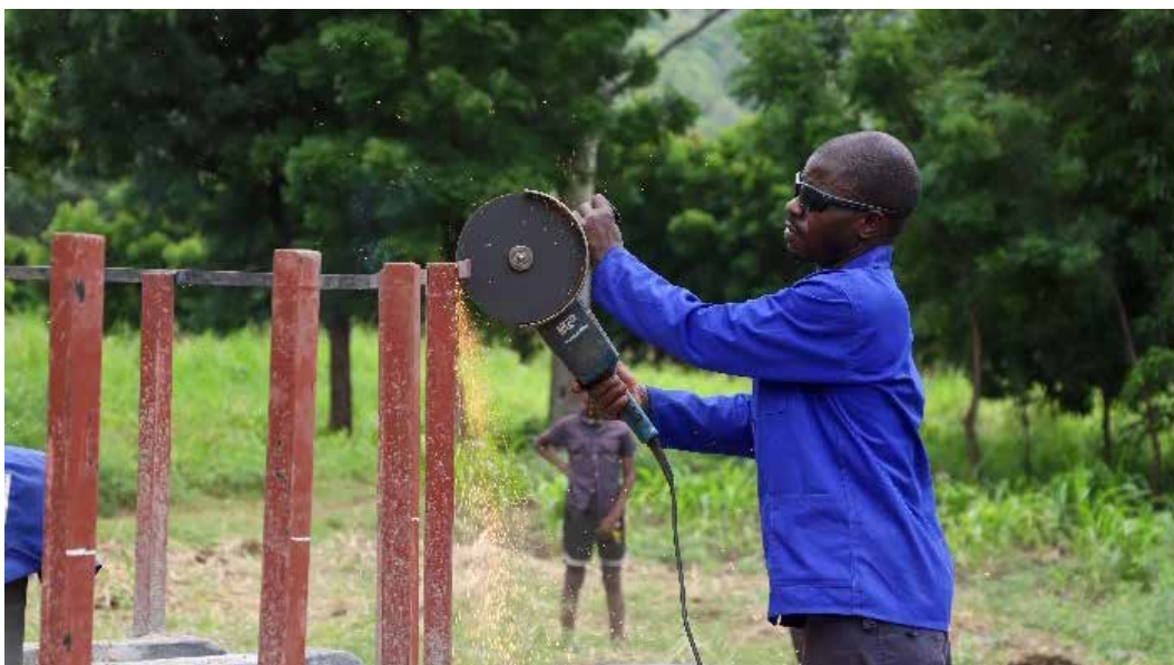
■ Figure 13: Welding of guard rail by certified welder
