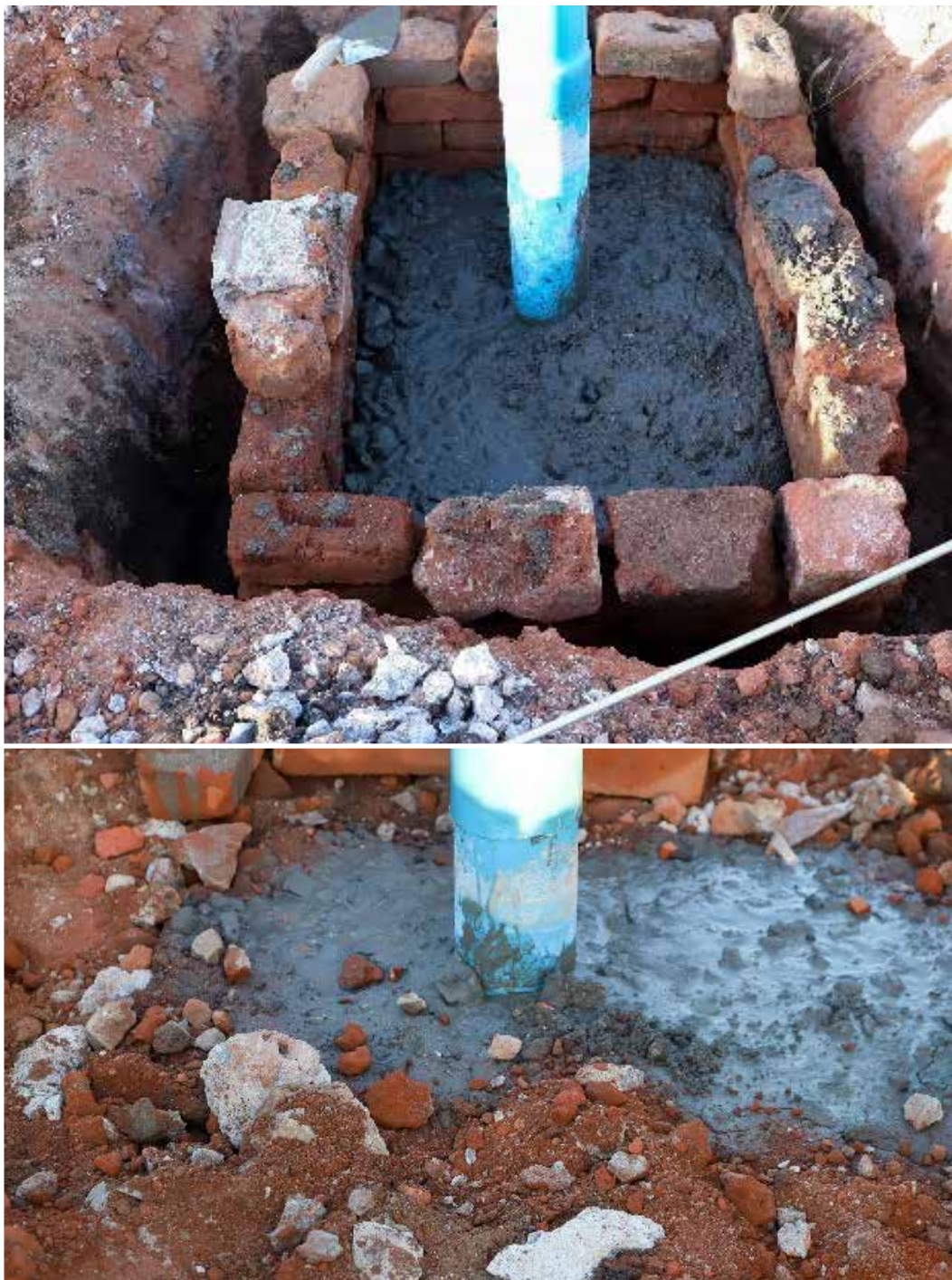
■ Figure 6: Concrete is poured around the base of the pump
