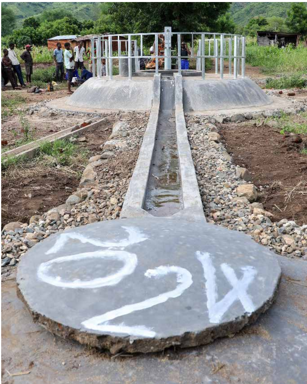
■ Figure 19: Flood proofed borehole
