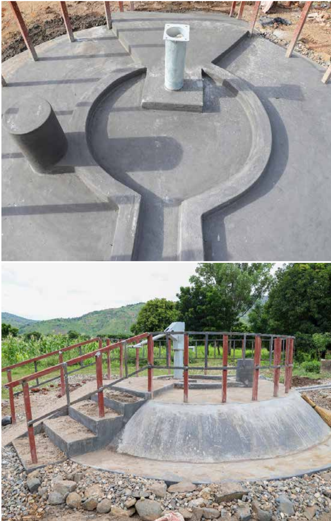
■ Figure 15: Finished platform and welded guard rail
