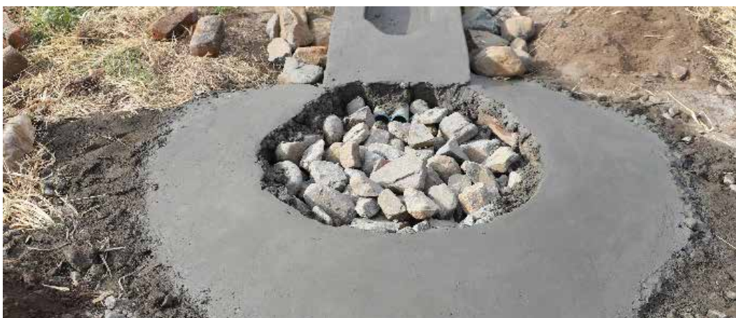
■ Figure 14: Drainage channel and soak pit filled with recommended stone aggregate
