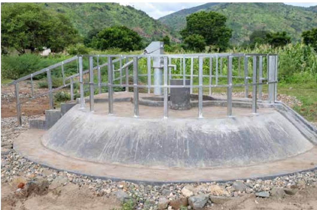
■ Figure 18: Finished flood proof borehole platform
