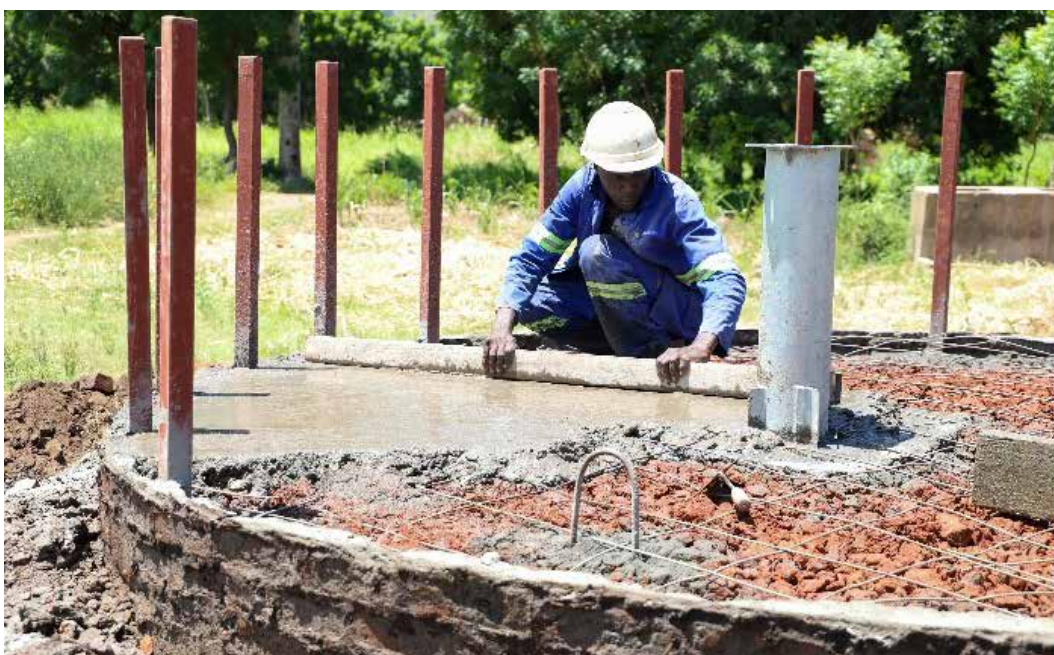
Figure 10: Reinforcement of the concrete platform base
