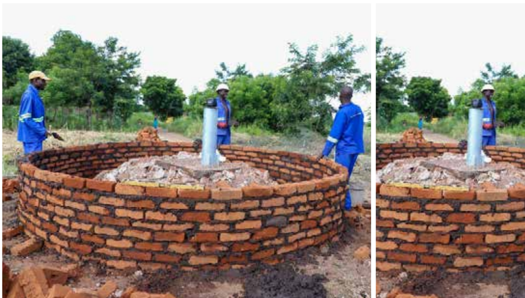
Figure 9: Construction of raised platform
