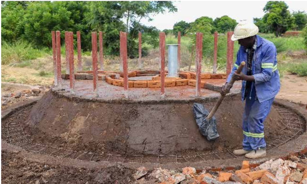
■ Figure 11: Construction and Reinforcement of second level of concrete platform base
