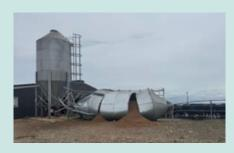
Feed silos may collapse if their structural integrity is compromised. This could be from a collision with a vehicle, from an earthquake, or from a lack of regular maintenance. Full feed silos can weigh more than 18 tonnes and could cause significant injury or death if they collapsed.
