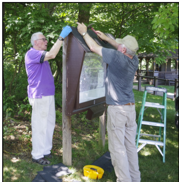
Herm Mast (left) and Grady Botens repairing the trail kiosk
