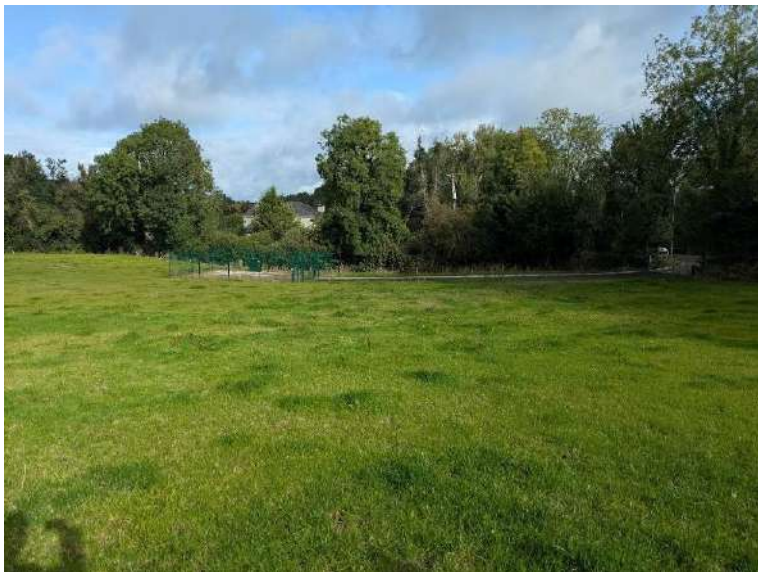
Plate 7: Pumping station in Field 1, facing north.
