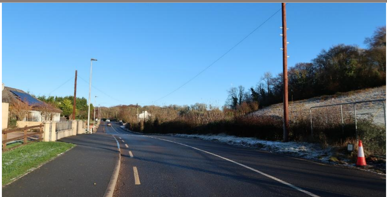
The Loreto Road (L1513) located to the north of the Application Site near the proposed site entrance.
